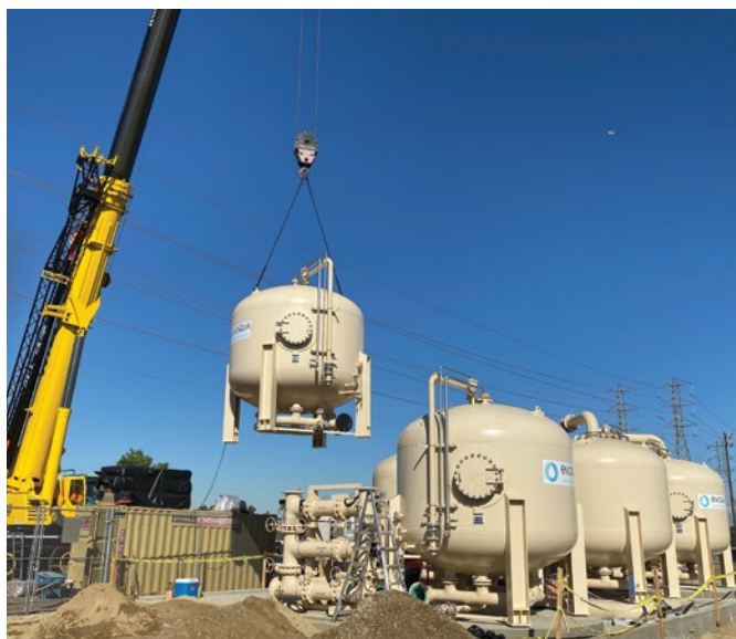
The Santa Clarita Valley Water Agency's new site near the William S Hart baseball and softball field in California was fast-tracked to treat 6,000 gallons per minute of PFAS-contaminated groundwater.
