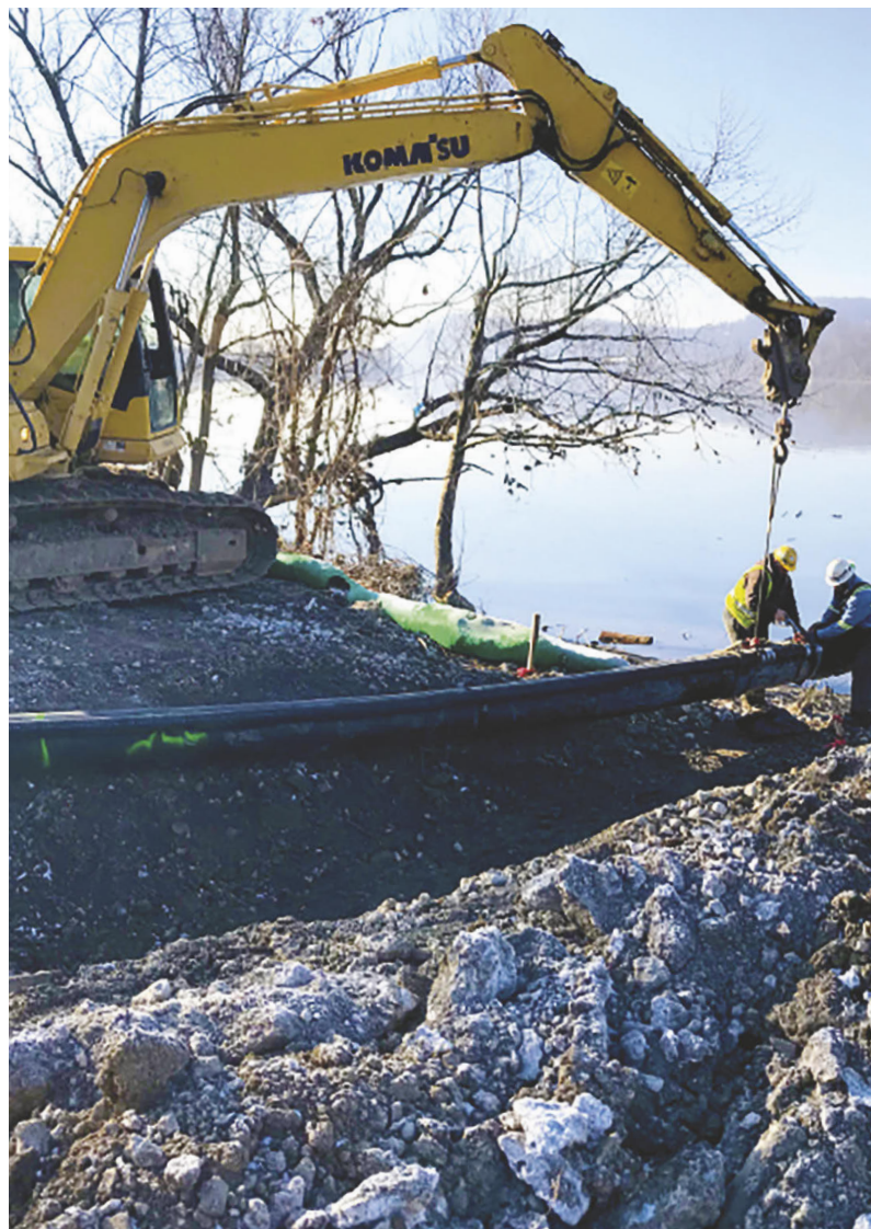
McKim & Creed furnished design-build services for a water intake facility, pump station, and pipeline (above) to transport water from the Ohio River via a freshwater pipeline. In terms of total megawatts installed (right), McKim & Creed has developed approximately 7 percent of the solar energy generation in North Carolina and Florida combined.
